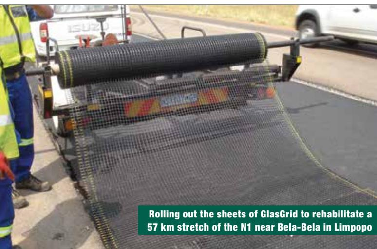
Rolling out the sheets of GlasGrid to rehabilitate a 57 km stretch of the N1 near Bela-Bela in Limpopo
