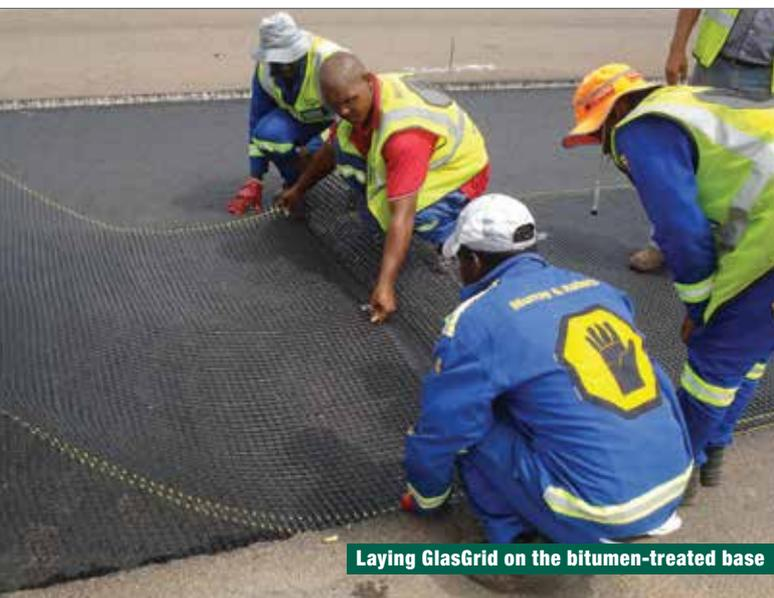
Laying GlasGrid on the bitumen-treated base
