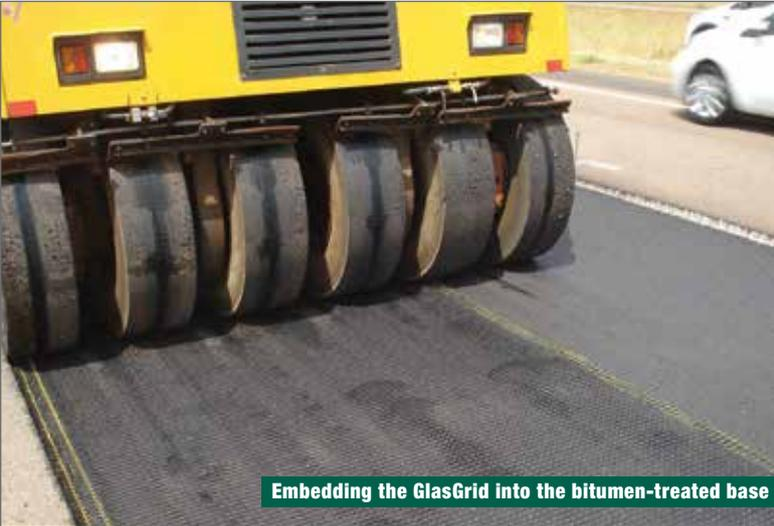
Embedding the GlasGrid into the bitumen-treated base
