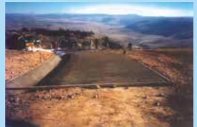
**Use sacrificial Hyson Cells BubbleLock™ formwork to cast articulated 3D interlocking cast-in-situ block paving with integral side-drains.**
