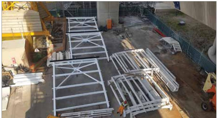
Figure 5: Structural steel roof segments ready for erection
