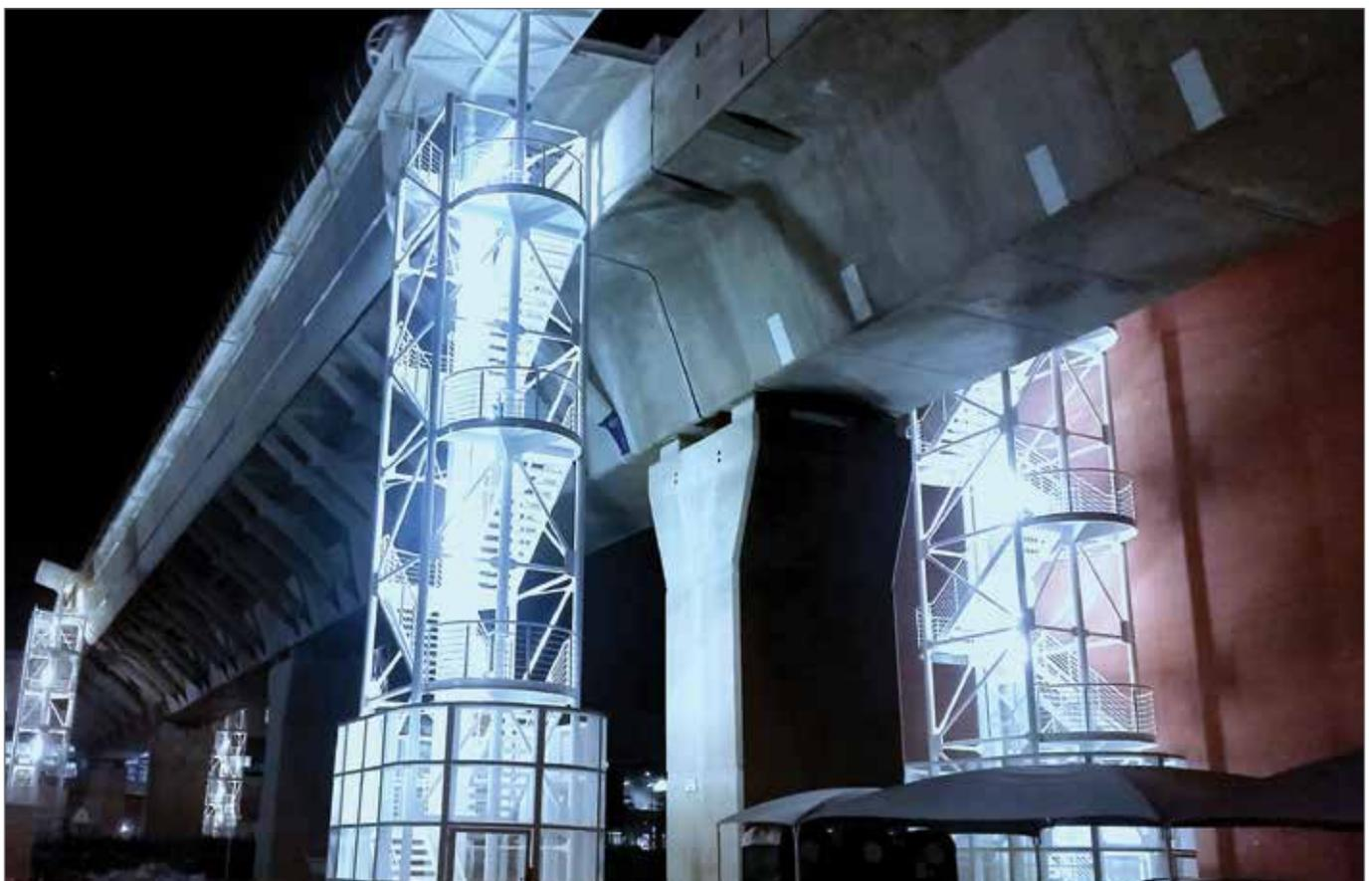
Figure 9: The completed viaduct structure with fire escape staircases as seen at night
