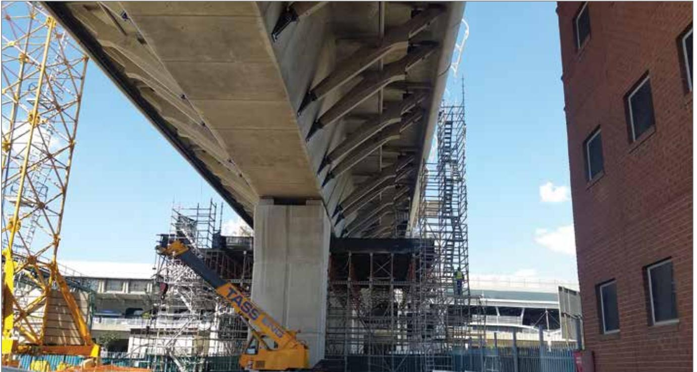
**Figure 7: Underside of the viaduct – this photo illustrates the new width of the station extension, as well as the temporary crash deck which is visible behind the mobile crane; the fixed crane is also partially visible to the left of the photo**
