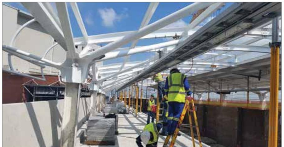
**Figure 3: Southern side roof construction during installation of sheeting and services**
