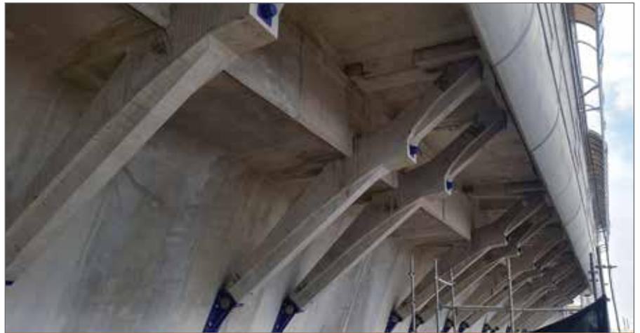
**Figure 2: Precast struts attached to the viaduct section**
