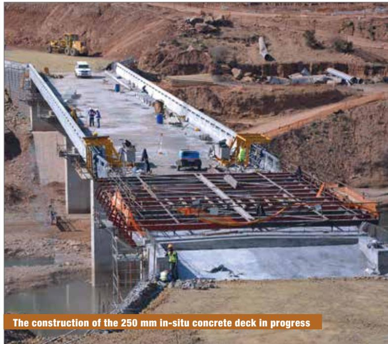
The construction of the 250 mm in-situ concrete deck in progress
