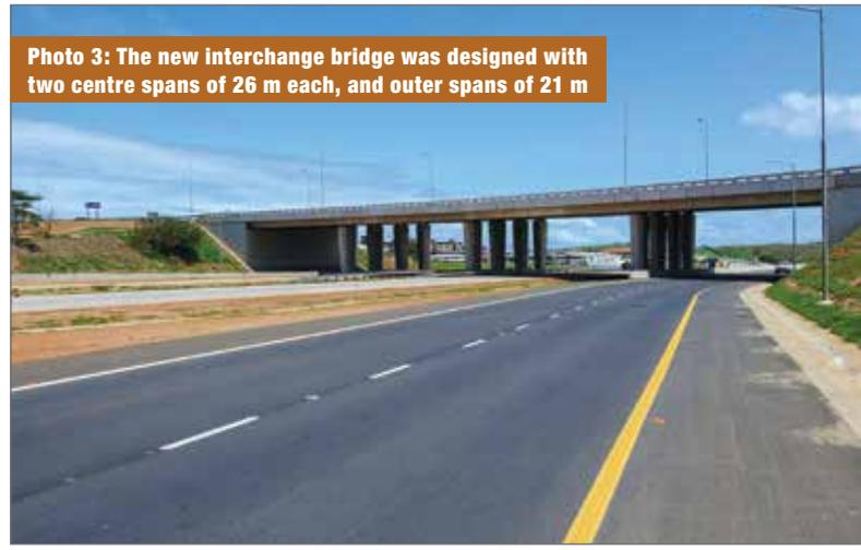
**Photo 3: The new interchange bridge was designed with two centre spans of 26 m each, and outer spans of 21 m**
