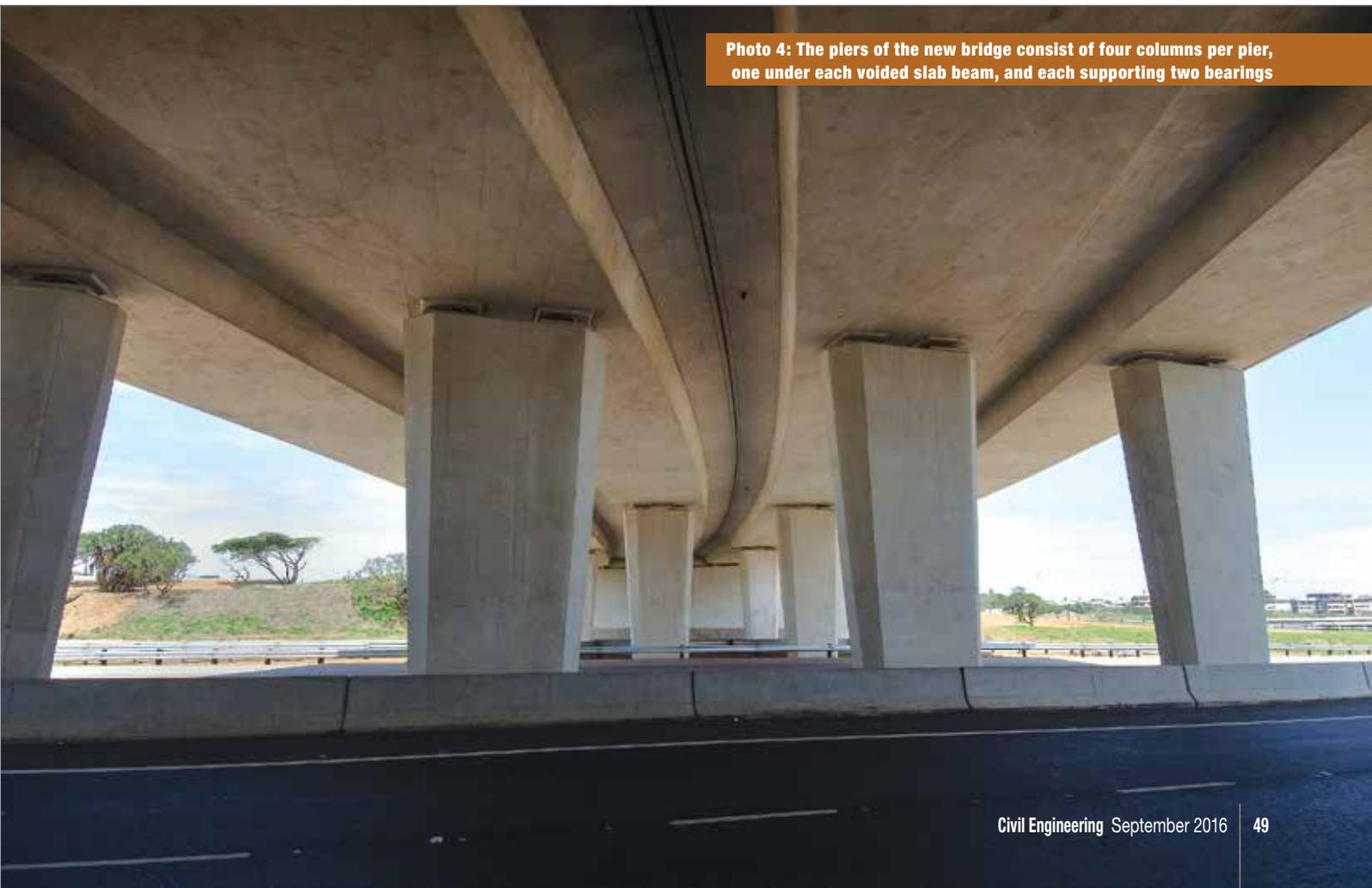
**Photo 4: The piers of the new bridge consist of four columns per pier, one under each voided slab beam, and each supporting two bearings**
